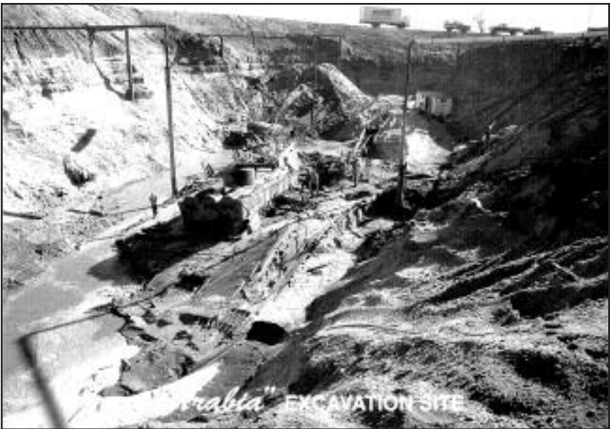
Excavation site beneath a Kansas corn field. Courtesy of Greg Hawley
