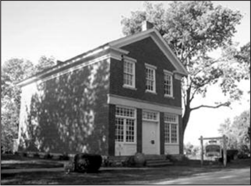
Joseph Smith's Red Brick Store, September 2001. Following the completion of the construction of the Red Brick Store in January 1842, meetings of the Nauvoo City Council and the municipal court were held in the building's second story. Photograph by Alexander L. Baugh.
